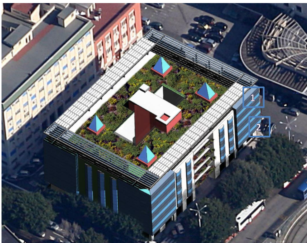
FIGURE 264 - AREAS AVAILABLE FOR THE PV SYSTEM INSTALLATION
