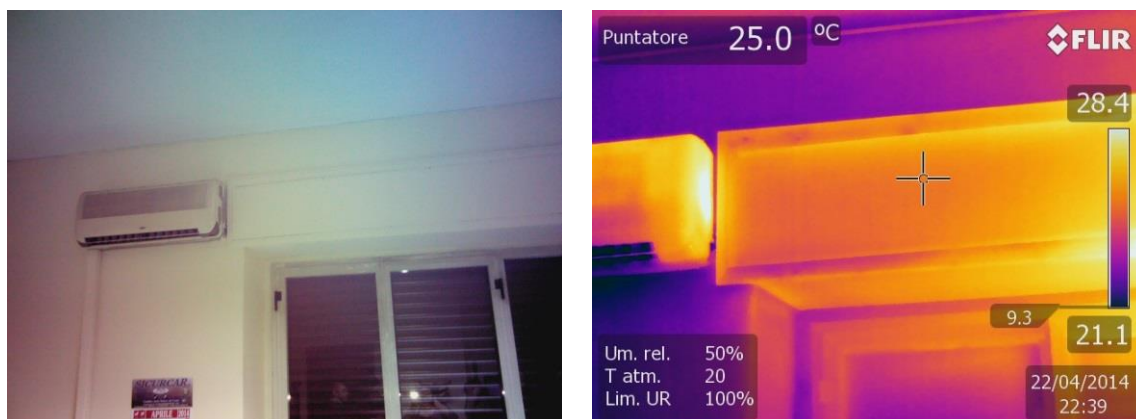
FIGURE 234 - THERMOGRAPHY OF AN AIR CONDITIONER ON
